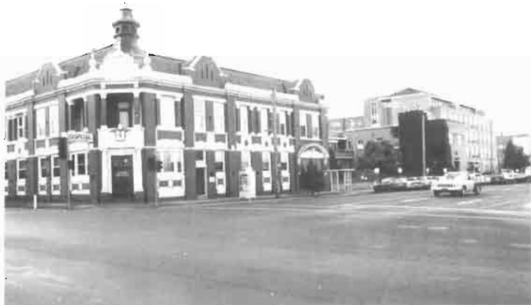
Outpatients Department and Administration Block, Ballarat Base Hospital.
