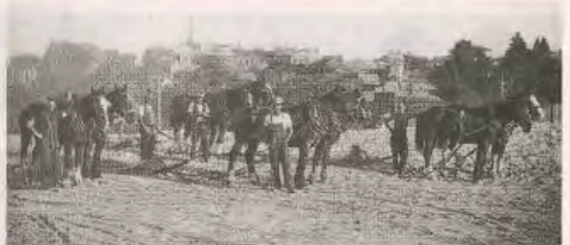
Preparation of new hospital site.
