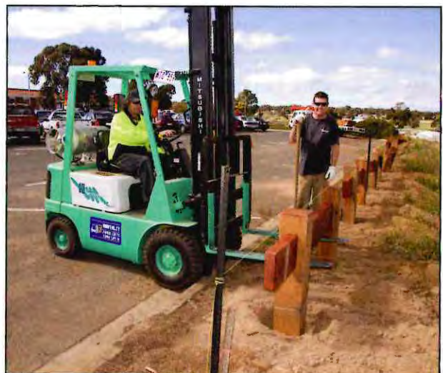
The new safety fence surrounding the helipad
