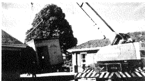
Crane operation during renovations to Radiology Department
