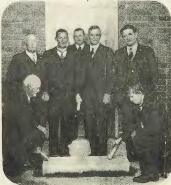
Messrs W. Harris and W. Campbell relaying at new Hospital Entrance the Foundation Stone of the Pleasant Creek Hospital on 12th December, 1933.
