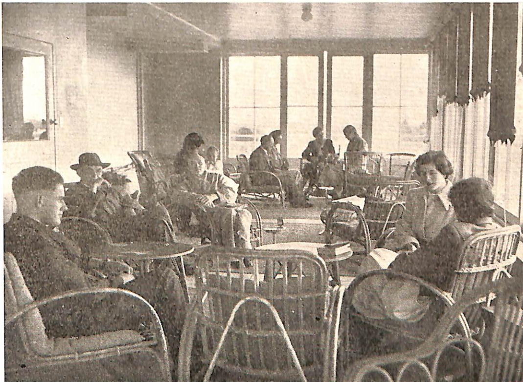
Solarium—First section of new hospital buildings
