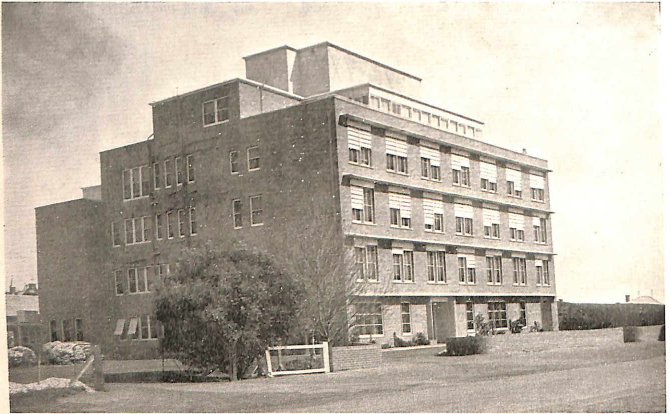
NEW BUILDINGS - - First Section Completed
