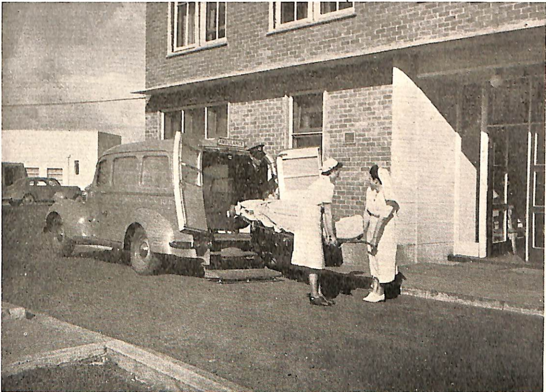
Ambulance discharging patient at front door of Hospital
