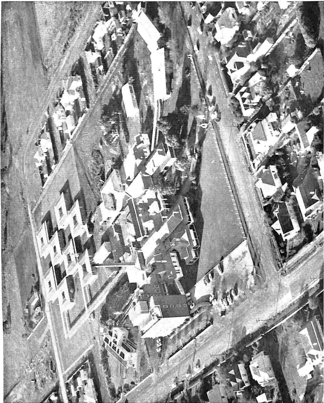
THE HOSPITAL FROM THE AIR, SHOWING COMPLETED NURSES' HOMES AT CENTRE REAR
