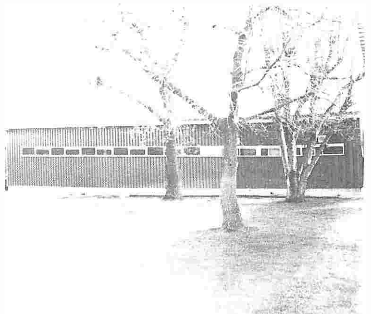
Building extensions to the Engineering Department
