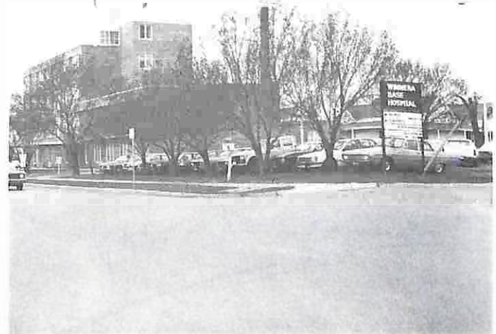
View of the main block of the hospital.
