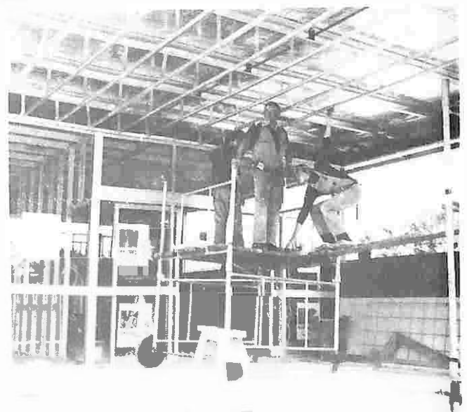
Tradesmen at work on the new hospital casualty entrance.
