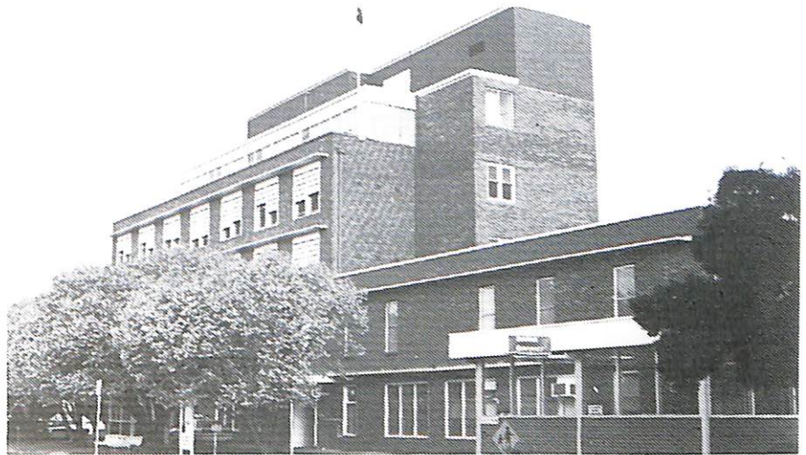
The existing Main Block Building will be refurbished to accommodate allied health and administration departments once the new acute facility is open.
