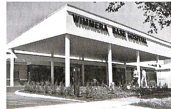
Right: The new acute hospital was officially opened on 24th April 1996 by the Premier of Victoria, the Hon. Jeff Kennett.
