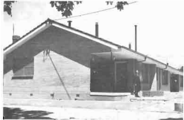
A view of the "Joe White Flats" erected in Windermere Street to meet accommodation needs of the hospital's senior professional staff.
